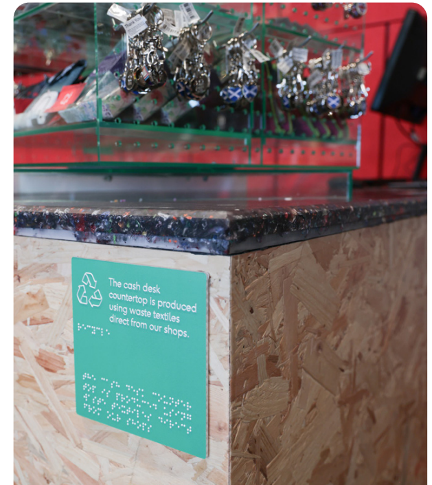
Shop countertop made from waste textiles
